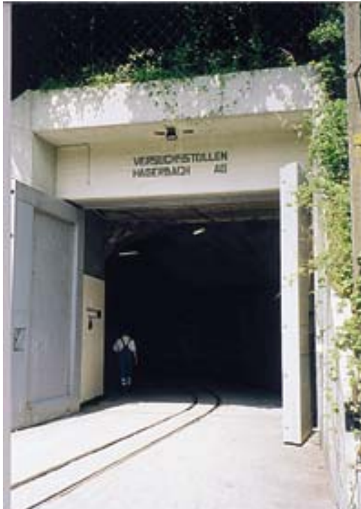
Entrance to the Hagerbach (Switzerland) test tunnel
