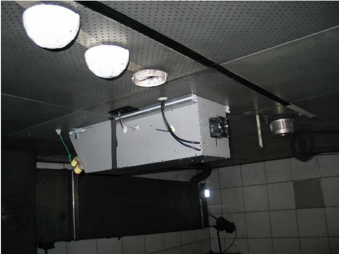
Figure 3: Photo of the prototype dry heat tunnel as mounted in the fire test room.
